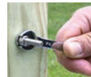
Tighten nut to tension
