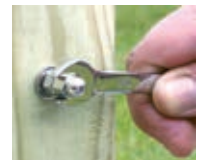
Cut thread leaving 1/4” and install acorn nut
