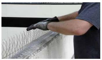
Stainless steel spike installed on rooftop parapet wall.
