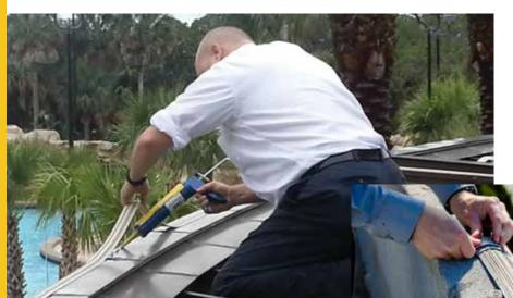
Bird Jolt Flat Track® easily glues in place with construction grade adhesives. Installation requires general knowledge of electrical systems. If you have questions or need an Authorized Installer call us at 800.392.6915.
