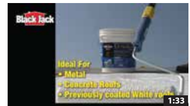
How To Prep a Roof and Apply Reflective Coatings
