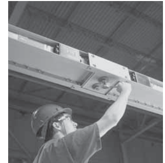
Typical Busway Installation (Torque Indicating Bolt)
