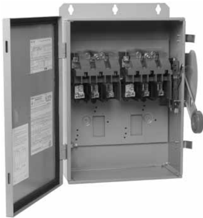
Six-Pole Motor Circuit
