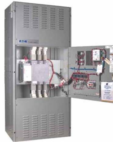
1600 ATS with ATC-300+ Controller
