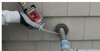
Around gas lines
