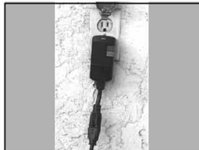
(H) Unplug the GFCI from the Power source.
