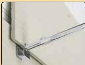
Depress thumb tab to allow plank to snap flush to wall and gauge.
