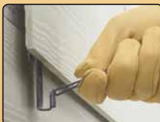
Remove gauge by depressing thumb tab again and lifting gauge up and off lower plank, then pulling gauge out from under top plank.
