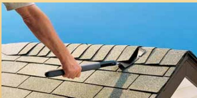
Handle those tight spots with a *short handled "Baby" BEAST!* For steep pitched roof caps and hard to get at dormers, overhangs, valley flashing and flashing around structures, this compact tool is indispensable. The short handled BEAST also features extra side slots for pulling out nails along walls and from under trim. One piece steel integral handle is covered with a comfortable foam grip.
