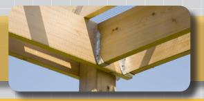
HOT DIPPED GALVANIZED PRODUCTS CONFORM TO ASTM A153
