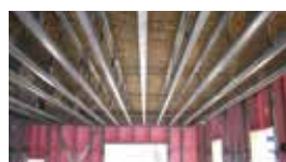
OSB and plywood to iSPAN joists
