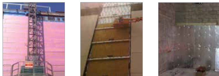
Exterior walls - Insulation to concrete
