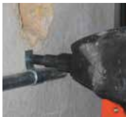
12HSMPO34 clip assembly used to secure conduit
