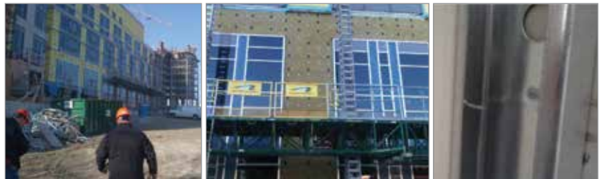
Exterior walls - Insulation to steel stud
