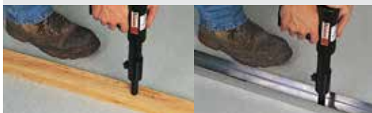
2" x 4" to concrete slab
