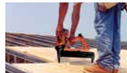
Plywood attachment—using TrakFast plywood to steel pin
