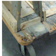
Wood—splinters and rots
