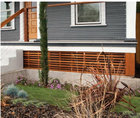
Panel Screen incorporated into porch design.
