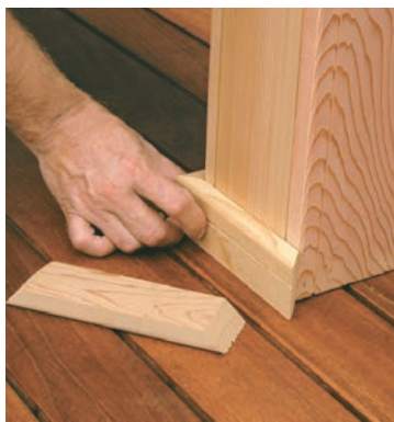
Assemble base moulding
