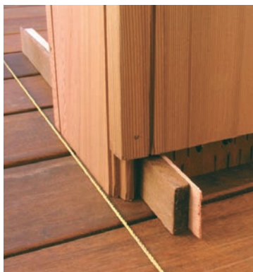
Shim bottom of post
